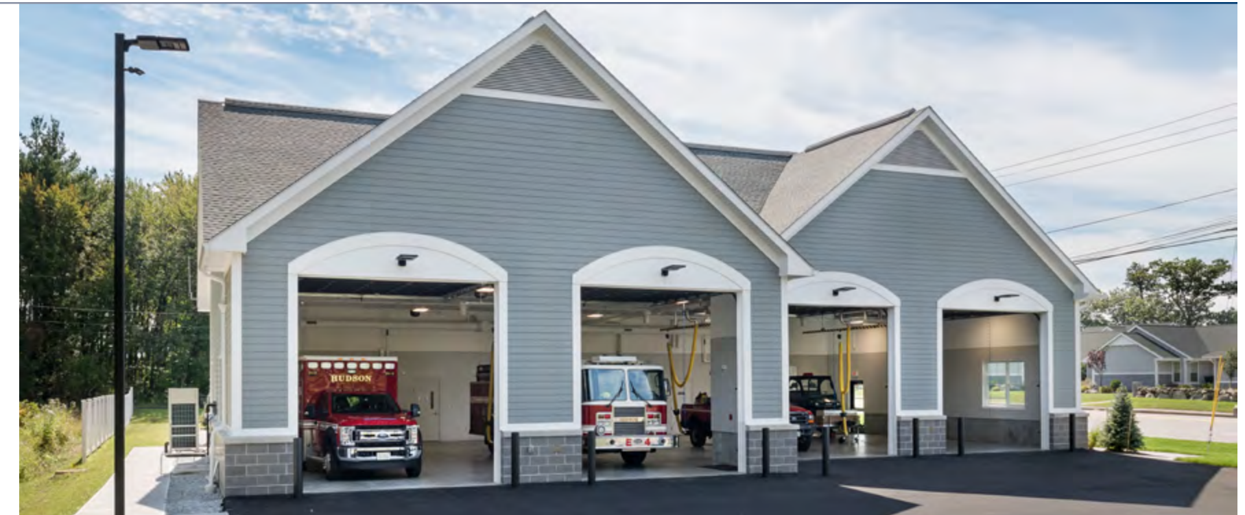
Above ▲ The fire station is the first new building the town has built in nearly 30 years
