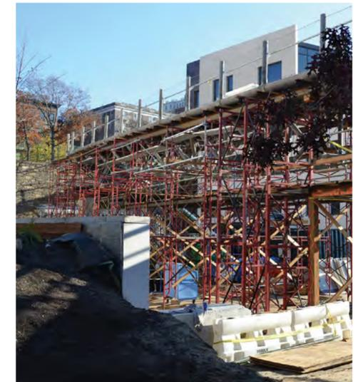
Above ▲ Adjustable scaffolding was used to support and reposition the bridge before connections were strengthened
