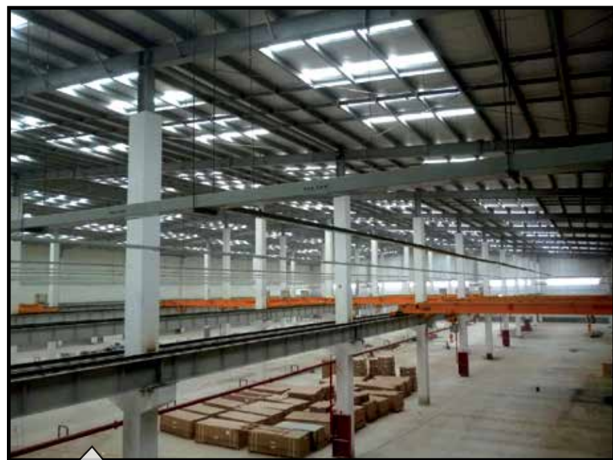
The consolidated manufacturing and distribution facility is in Xian, China.
