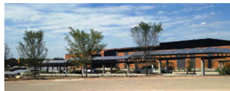
Above ▲ North side view of the new data center
