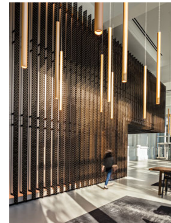
▼ Below Each aluminum panel was fabricated and installed individually
